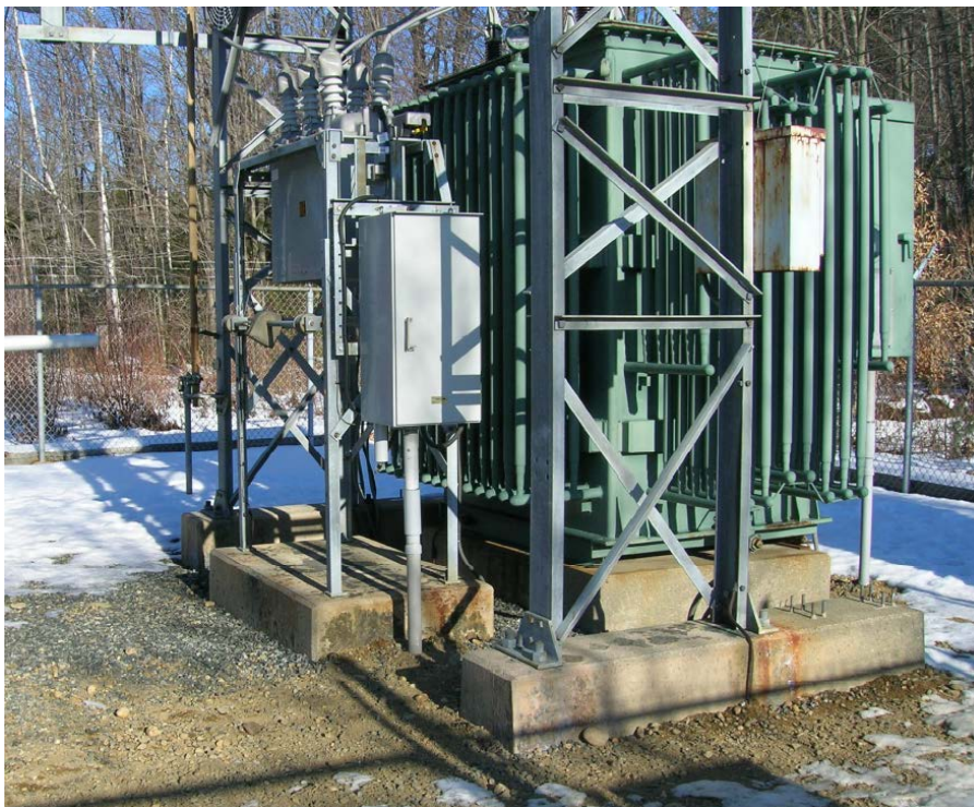
Existing Three Phase Regulator at East Northwood SS
